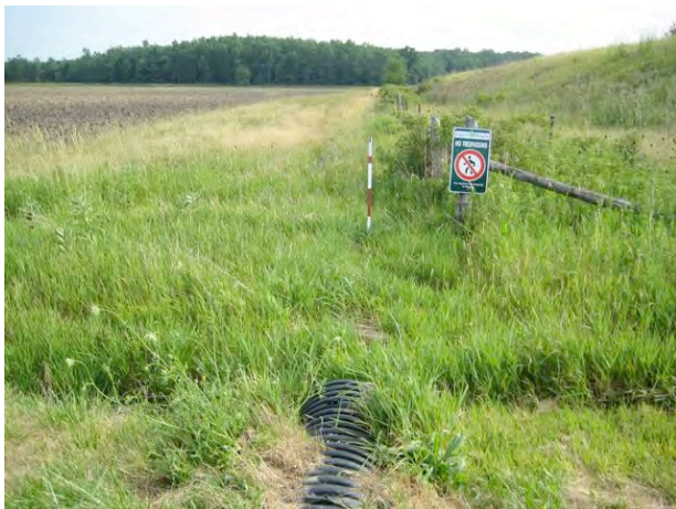
Figure 3: Another view of north-south unnamed drainage located immediately west of Subject Lands.
